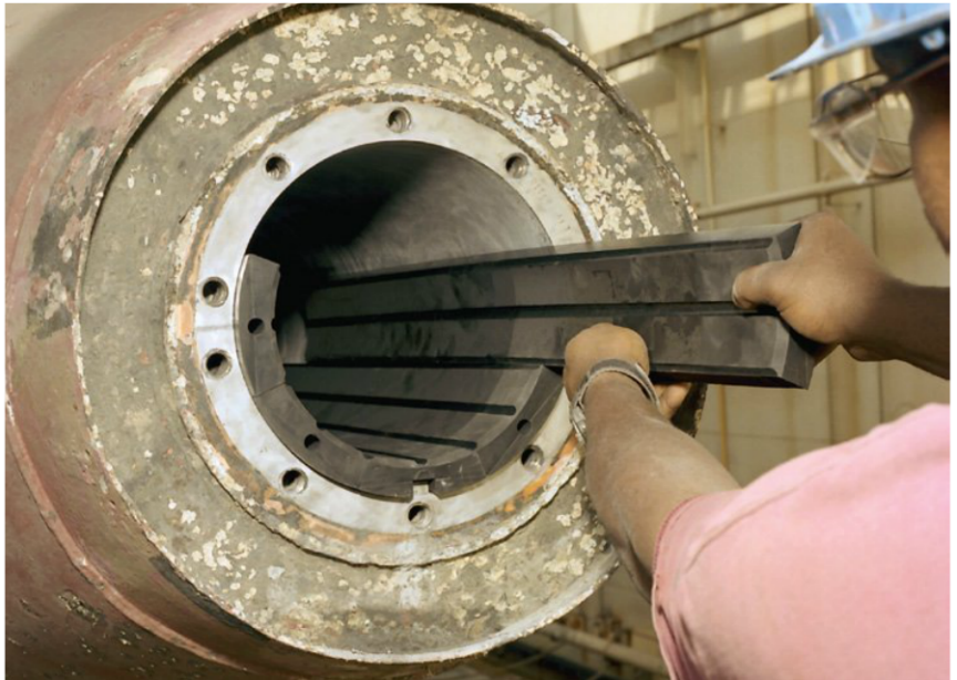
Fitting rubber staves into an existing housing tube
